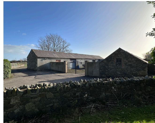
Entrance to the courtyard
